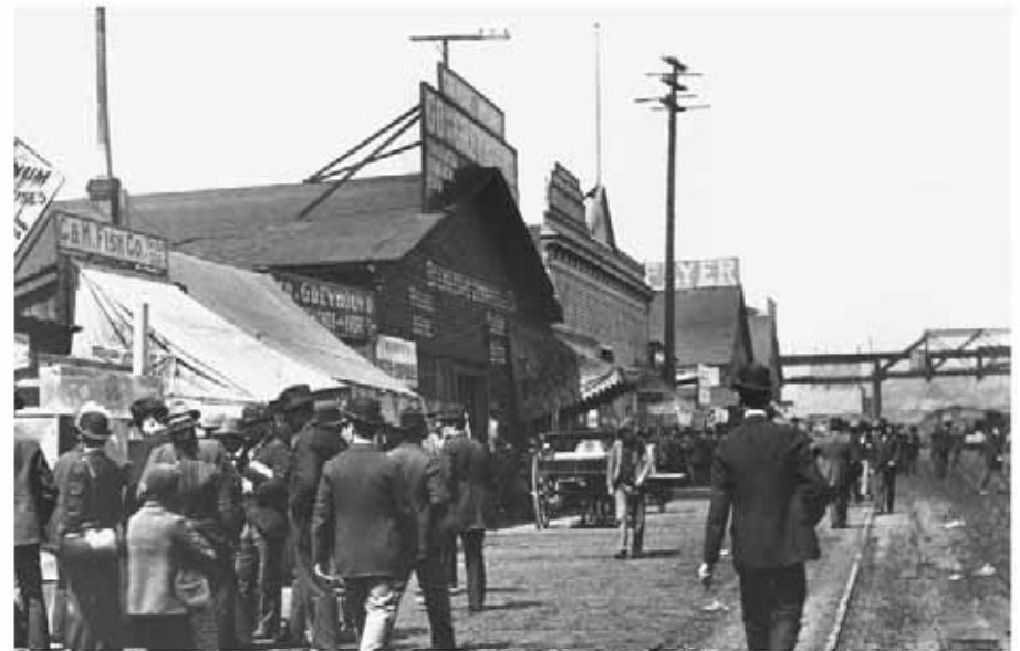
Colman Dock, left, and Marion Street trestle bridge, right, ca. 1909. Courtesy of Paul Dorpat
