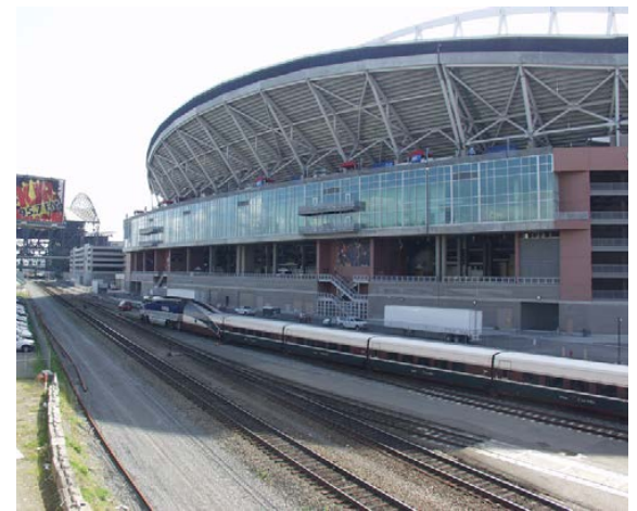
overtracks site east of CenturyLink Field
