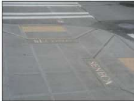
Accessible ramps in the central business district
