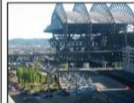
Traffic accessing 4th Ave S
