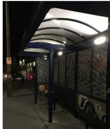
Internal lights are of various types, some lighting the roof, others lighting glass patterns - all are direct view and have significant glare.
